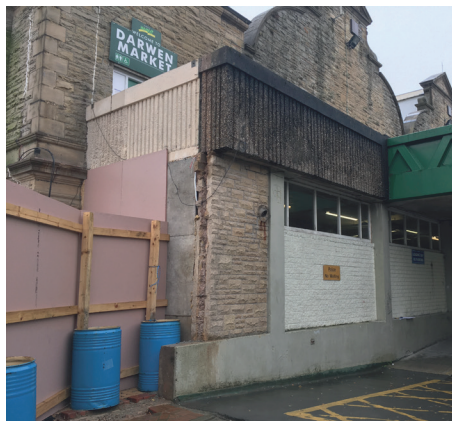
Existing boarded up entrance
